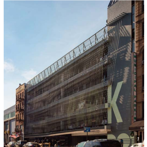
Figure 1. The Delancey and Essex Municipal Parking Garage showing the woven façade © Paul Warchol Photography
