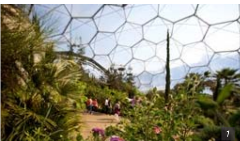
Figure 1. Eden Project (Garden of Eden), St. Austell, UK, architects: Sir Nicolas Grimshaw & Partners, structural engineer: Anthony Hunt & Associates, execution (ETFE-Foil cushion structure): Vector Foiltec © Vector Foiltec
